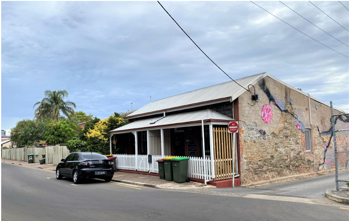
Photo 1 – The front of the site
