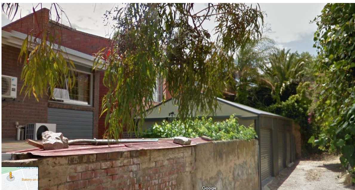
Figure 2: Rear of subject land (partially obscured by vegetation) and grey garage to be replaced.
