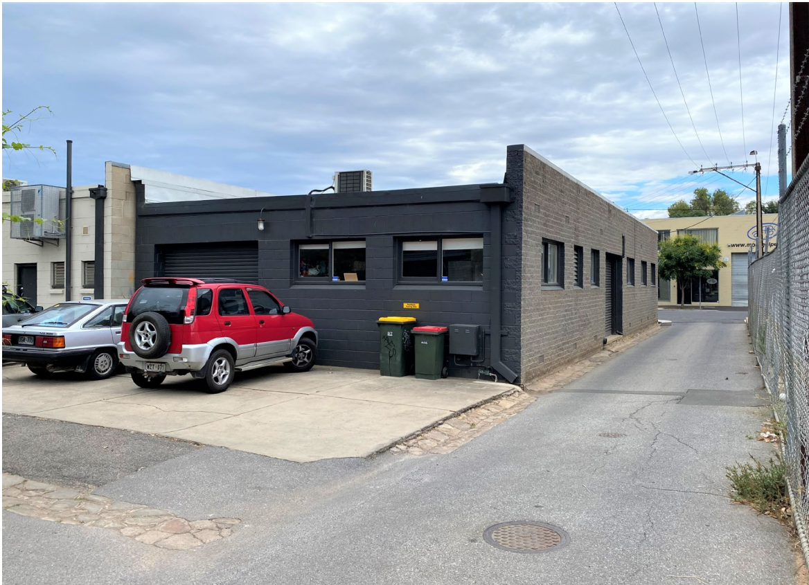
Photo 3 – The rear of 263 and 265 Gilbert Street which lie to the north of the site
